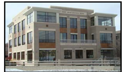
The office/professional services category occupies less than 1 percent of the County on the 2035 land use plan map. This category includes a variety of business uses and limited retail uses.
