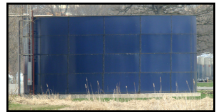
A manure storage facility. Reducing the human and environmental risks posed by animal waste is a goal outlined in Washington County's Land and Water Resources Management Plan.
