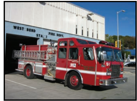
Washington County should encourage intergovernmental cooperation when selecting sites for locating public facilities such as fire stations.
